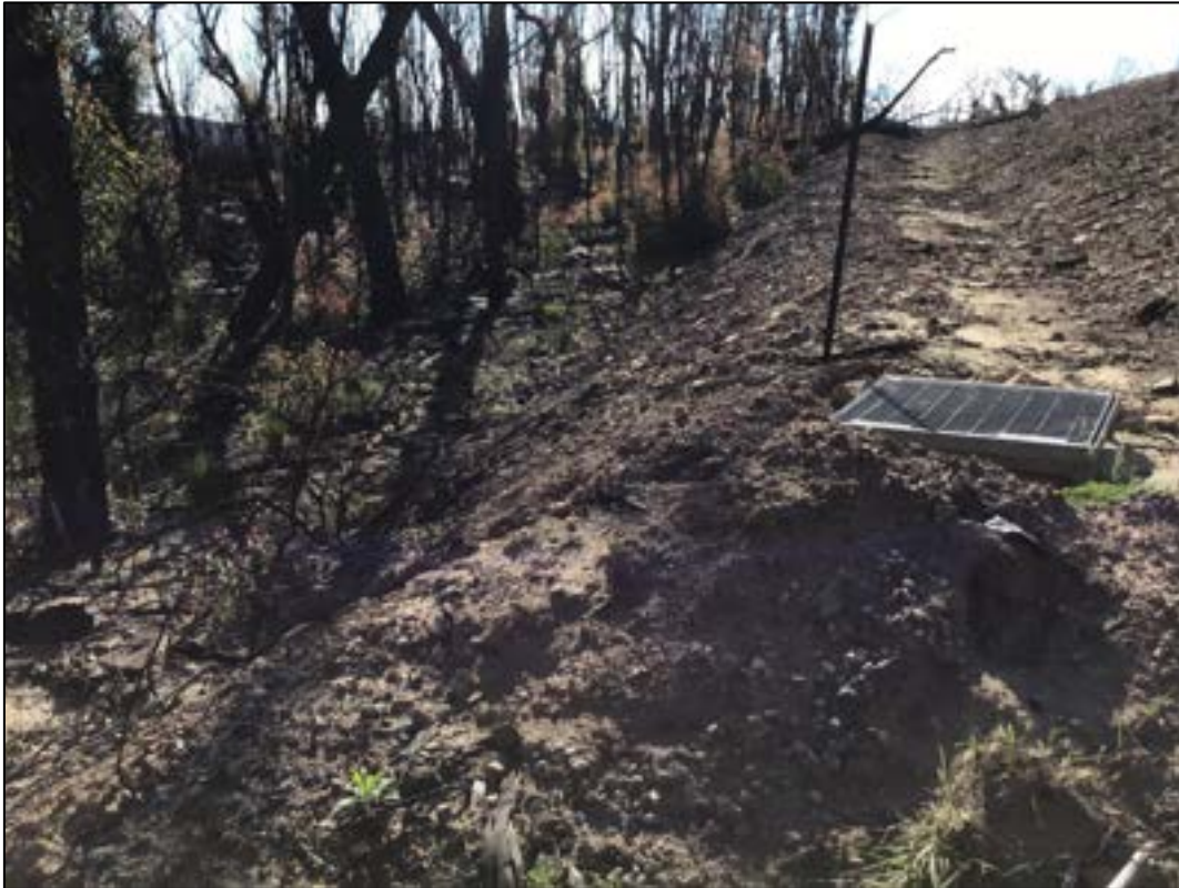
Plate 12. The character of the drainage pit and vegetation at the south-east corner of the 50 m gun range (date taken: 28/09/20).
