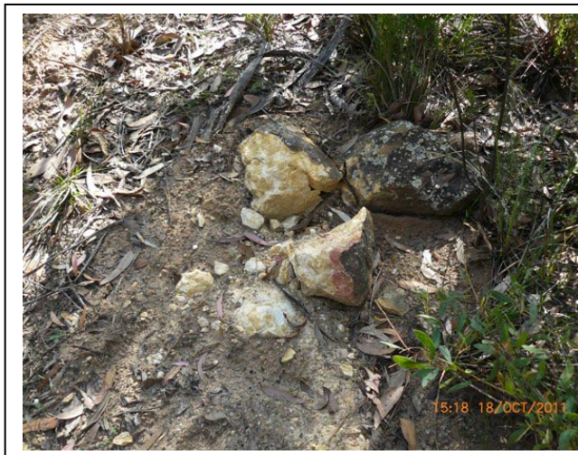
Broken rock on side of track
