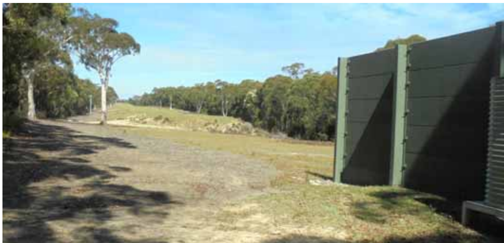
Images 2-4 Eastern Club House and portable Complex Office, Amenities building and the 800m Shooting Range
